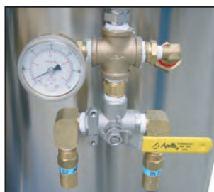
Dual Relief Valve Assembly
